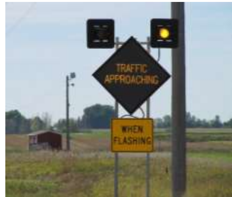
Photo: Minnesota Department of Transportation
