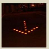
Raised Pavement Marker (RPM) Arrows at Exit Ramp (Source: Ouyang, 2013)
