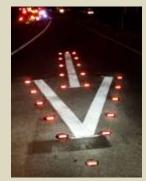
Raised Pavement Markers (RPMs) at Exit Ramp (Source: Provided by Arizona DOT)
