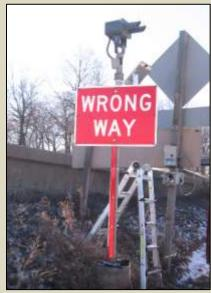
Ramp Detection with Camera for Verification at Exit Ramp (Source: Provided by Wisconsin DOT)
