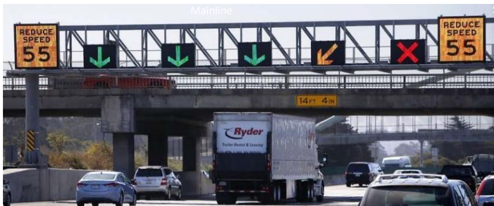
Figure 1: ATM Lane Use Control Signage on I-80 in the San Francisco Bay Area (Source: Caltrans)
