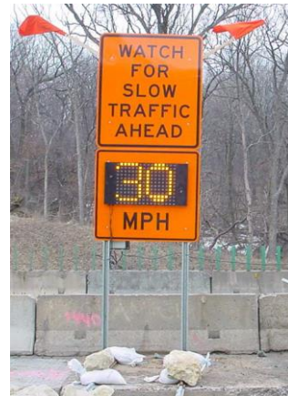
VSL Sign installed near Hwy 61 in Minnesota
