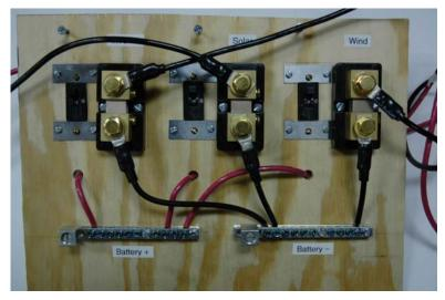
Figure 21: Shunt panel.
