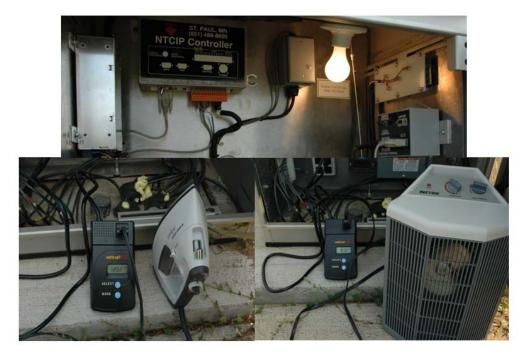
Figure 35: High load test using an iron, heater, and 100 watt bulb
