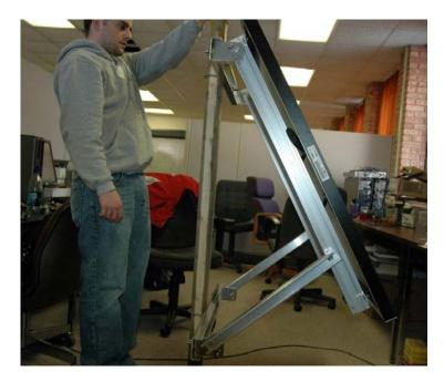
8. Adjust the tilt angle of the PV and the face direction as shown below. Tighten all nuts and bolts.
