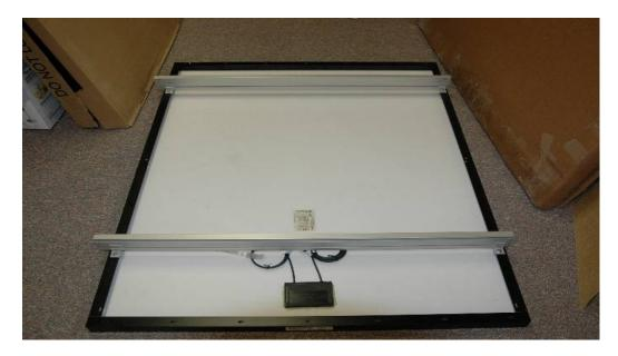
2. Tighten the clips using the 7/16" bolts, washer, and lock nuts.
