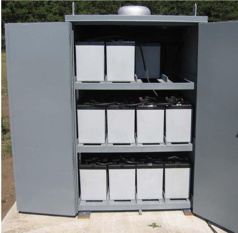
**Figure 19: Battery cabinet with 32 batteries.**
