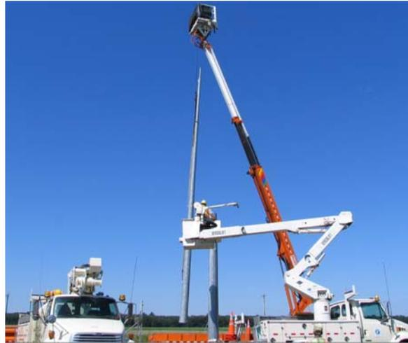
**Figure 22: Installation of the pole.**
