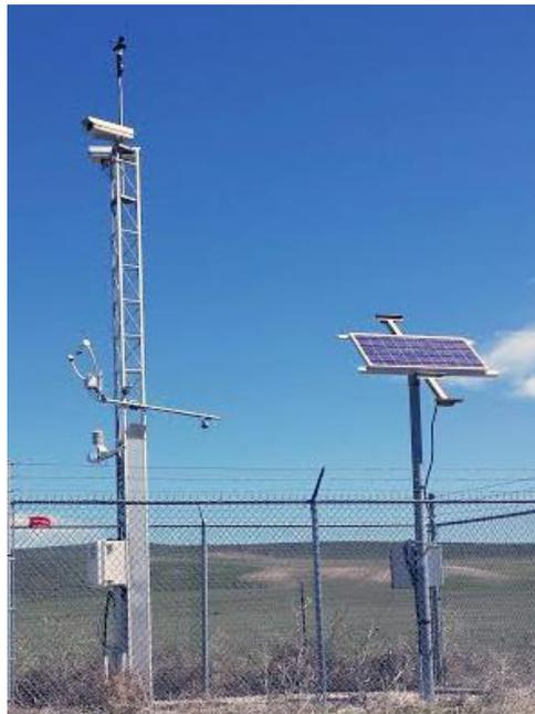
**Figure 3-7 Typical road weather information system deployment (Source: Campbell Scientific)**
