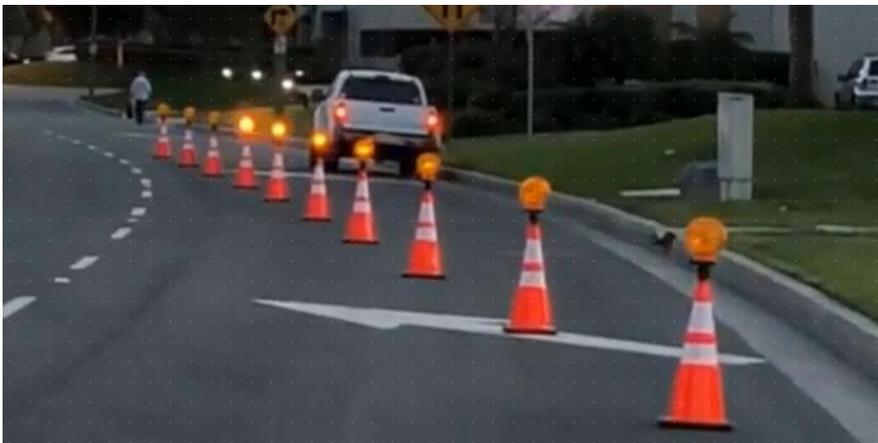
**Figure 3-1 Pi-lit Sequential Warning Lights (Source: Iowa DOT)**
