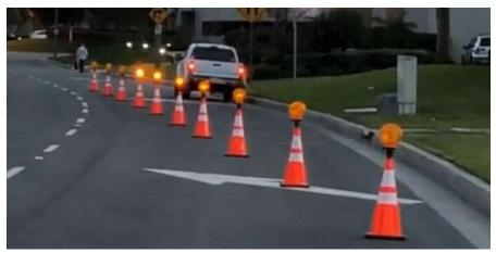
Figure 3-1 Pi-lit Sequential Warning Lights (Source: Iowa DOT)
