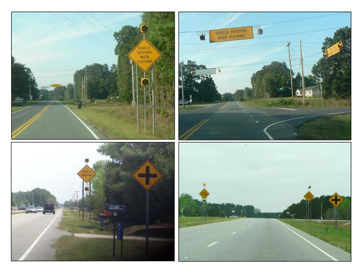
Figure 5: Photos of Mainline ICWS Deployment in North Carolina
