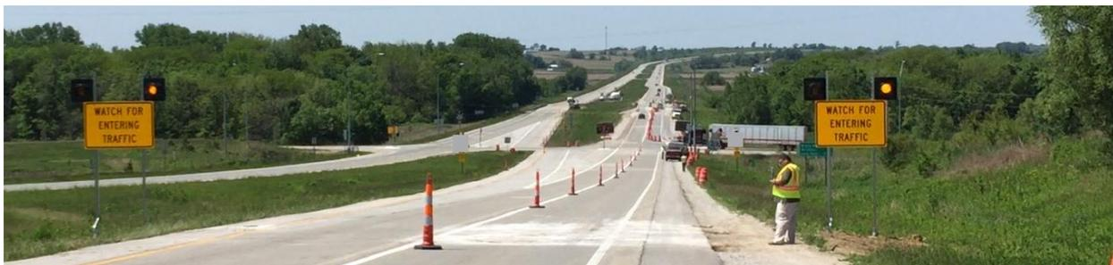
**Figure 3: ICWS Deployment for Mainline Traffic in Iowa**
