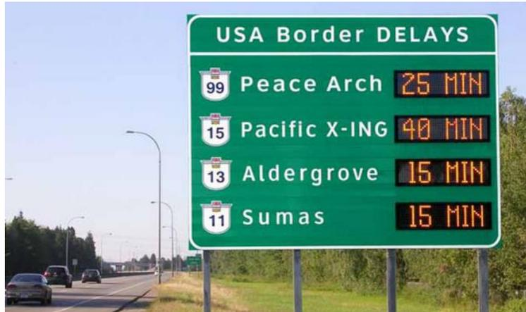
**Figure 4: Dynamic Message Sign Showing Border Delays**
