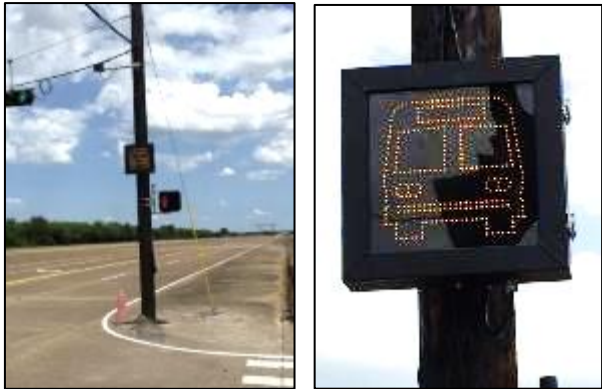
Figure 25: Supplemental bus alert signs at the intersection (Source: TTI)
