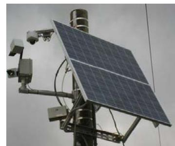
Figure 2-6 Solar Planes and Pole Mounted
