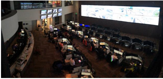
Figure 8: Remodeled San Antonio TMC March 3, 2021 Photo Courtesy of TxDOT
