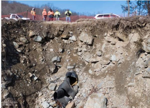
Figure 4.6 Screenshot of Drone Footage – Rockfall along I-287 (Source: [Innovation Spotlight: NJDOT UAS Program](#))
