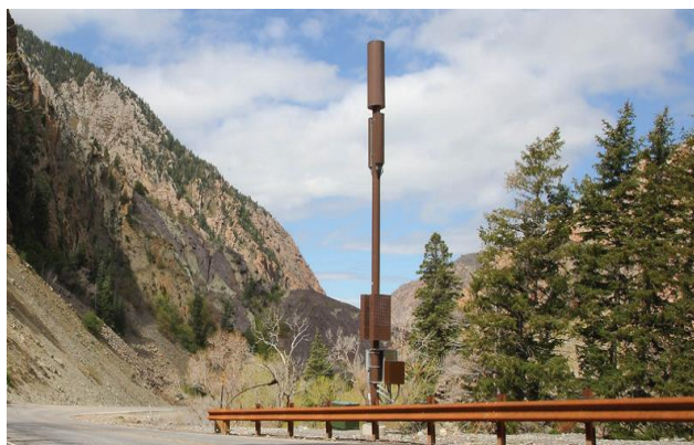
Figure 6: Distributed antenna system in Cottonwood Canyon, Utah (Source: Utah DOT)
