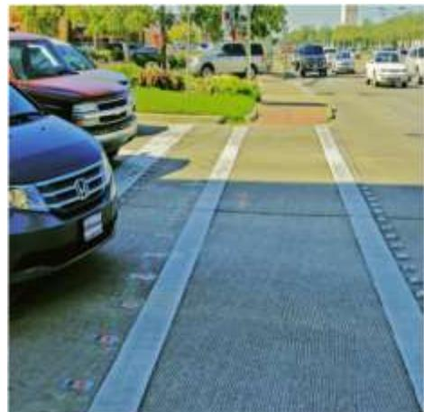
In-pavement LED Lighting at Exit Ramp
