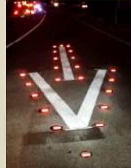
**Raised Pavement Markers (RPMs) at Exit Ramp**
