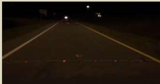
**Internally Illuminated Raised Pavement Markers Create Illusion of Stop Bar**
