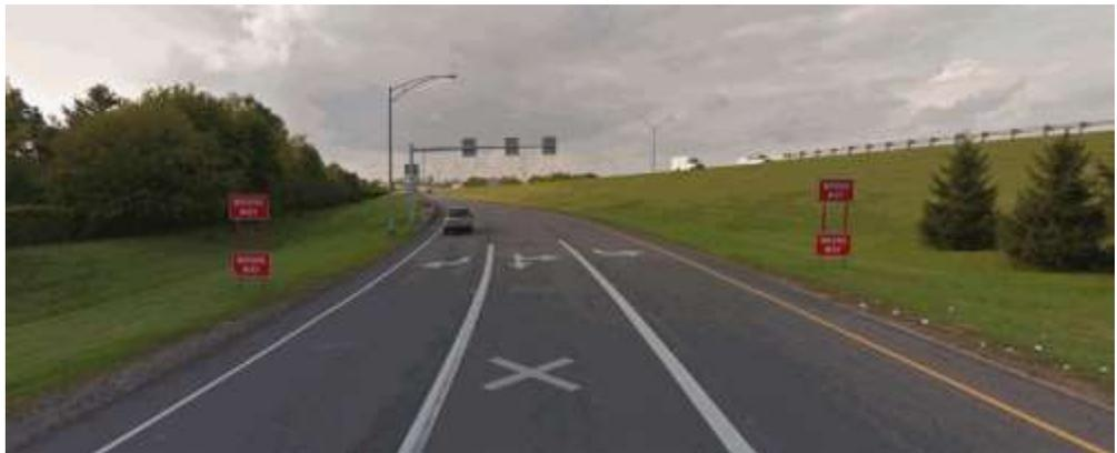
Two WW Signs on Same Post, Both Sides of Ramp, Red Reflective Tape on Posts
