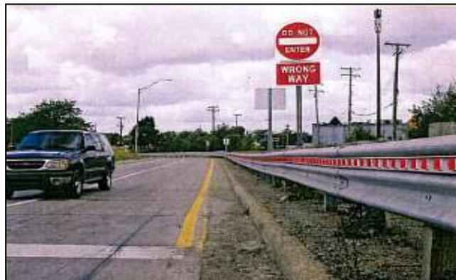
Red Delineators on Guardrail along Exit Ramp
