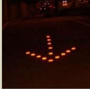
**Raised Pavement Marker (RPM) Arrows at Exit Ramp**
