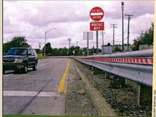
**Red Delineators on Guardrail along Exit Ramp**
