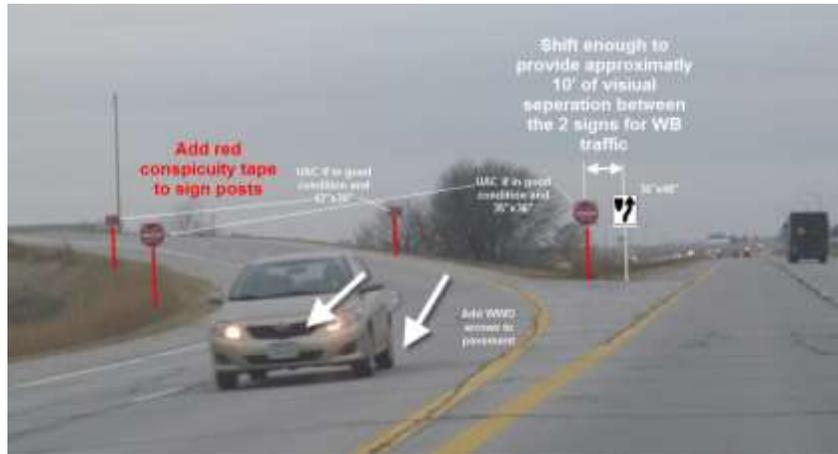
Improvements at Lincoln Way Flyover Ramp: Signs on Both Sides of Ramp, Red Conspicuity Tape on Posts, Wrong-Way Arrows
