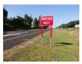
Oversized WRONG WAY Sign with Red Delineator Strips on Posts (Source: Connecticut DOT)
