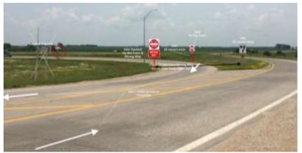
Improvements at 19<sup>th</sup> Street Interchange: Stacked DNE and WW Signs on Both Sides, Red Conspicuity Tape on Posts, Wrong-Way Arrows (Source: Iowa DOT)
