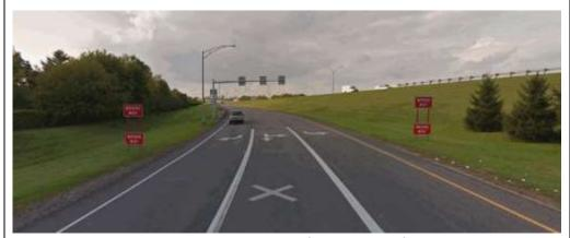
Two WW Signs on Same Post, Both Sides of Ramp, Red Reflective Tape on Posts (Source: Ohio DOT)
