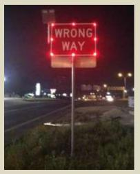
LEDs at WRONG WAY Sign Border, Flash Continuously at Night & Low Light (Source: Provided by Texas DOT)
