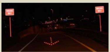
Red Reflective Tape on Sign Posts, Signs on Both Sides of Ramp (Source: Ouyang, 2013)
