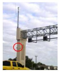
Radar Detection on Mainlane Mounted to Sign Bridge (Source: Texas DOT)
