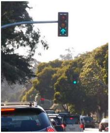
Straight Arrow Signal Indication to Discourage Turns onto Exit Ramp (Source: Rhode Island DOT)
