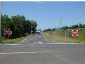
Oversized, Lower Height Signs on Both Sides of Ramp (Source: Connecticut DOT)
