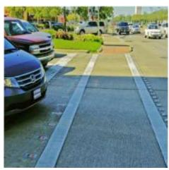
In-pavement LED Lighting at Exit Ramp (Source: Provided by HCTRA)
