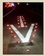
Raised Pavement Markers (RPMs) at Exit Ramp
