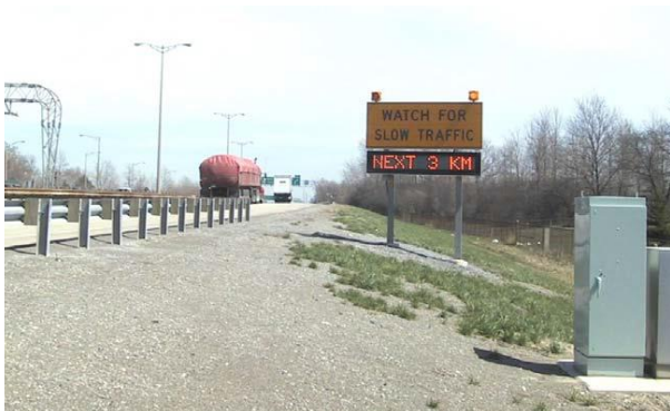
Figure 8: Queue Warning System Site in Ontario, Canada
