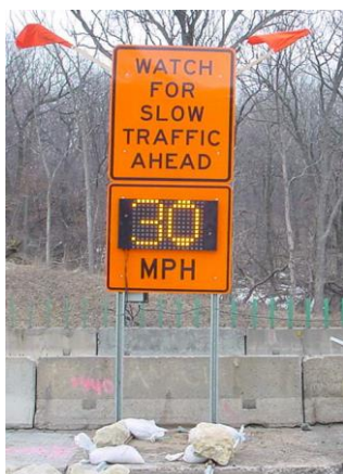
Figure 12: VSL Sign installed near Hwy 61 in Minnesota
