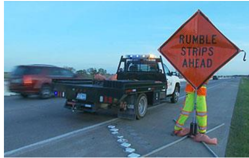
Figure 10: Queue Warning System in Texas Incorporates Temporary Rumble Strips 46
