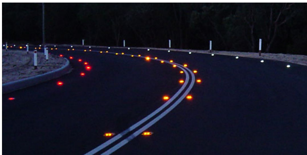
Figure 9 Example Application of LED Raised Pavement Markers.
