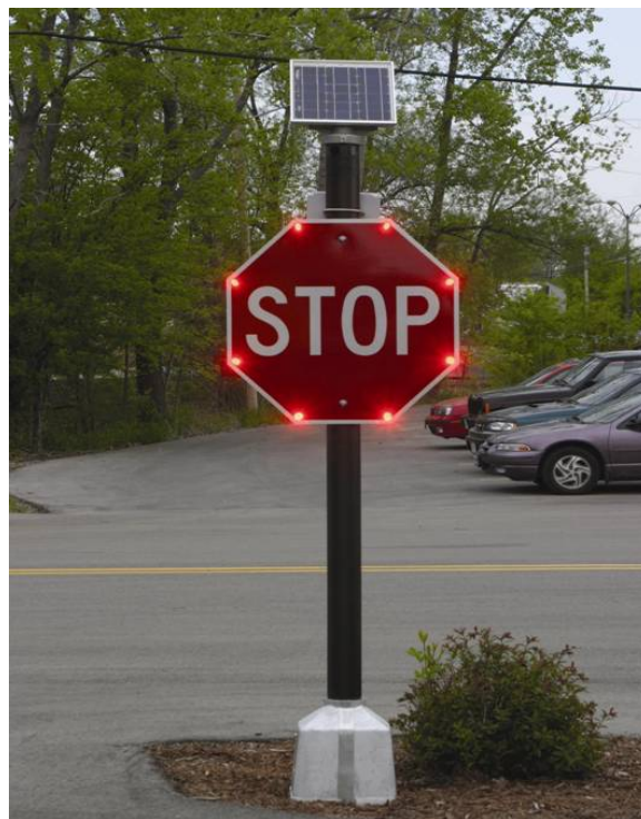
Figure 11 Example LED STOP Sign
