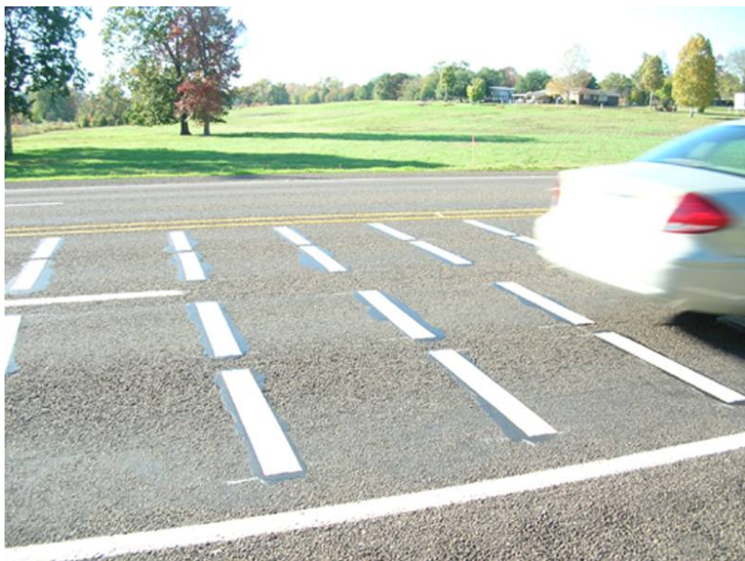
Figure 21 Thermoplastic Transverse Rumble Strips
