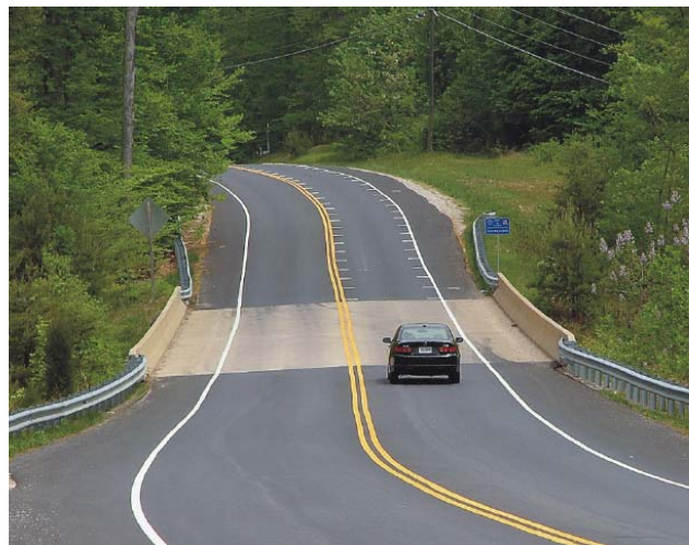
Source: Virginia Transportation Research Council
