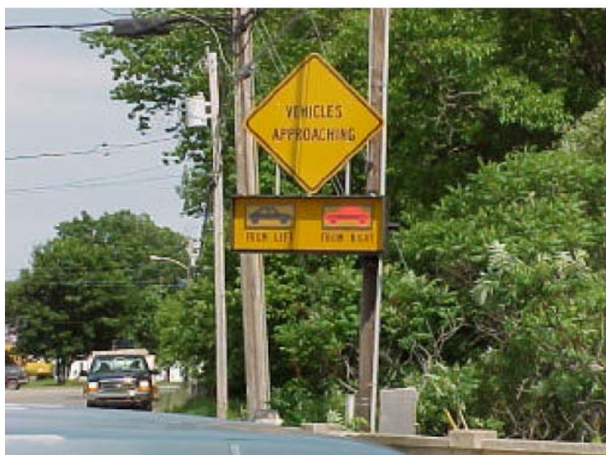
Figure 18 Vehicle Actuated Warning System (Norridgewock, Maine)
