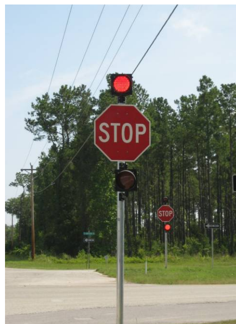
Figure 12 Example Vehicle Actuated Flashing Beacons
