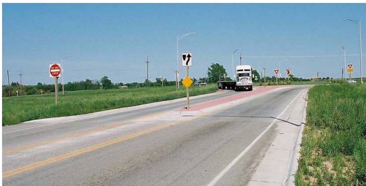
Figure 39 Extended Splitter Island on Rural Roundabout Approach (Kansas)
