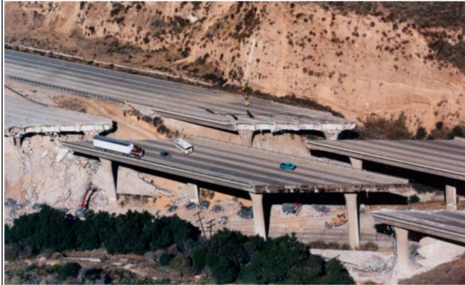
**Figure 1-2: Damage from Northridge Earthquake**
